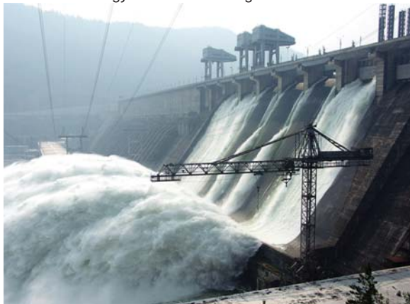
Figure 7.37 Hydroelectric facility (credit: Denis Belevich, Wikimedia Commons)
