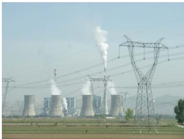
Figure 7.24 Tremendous amounts of electric power are generated by coal-fired power plants such as this one in China, but an even larger amount of power goes into heat transfer to the surroundings. The large cooling towers here are needed to transfer heat as rapidly as it is produced. The transfer of heat is not unique to coal plants but is an unavoidable consequence of generating electric power from any fuel—nuclear, coal, oil, natural gas, or the like. (credit: Kleinolive, Wikimedia Commons)
